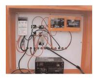
Power for the Smart Zone system is provided by 32 6-Vdc deep-cycle batteries connected in series-parallel. Additional power is supplied by eight 75-watt solar panels which can be directed toward the sun.
